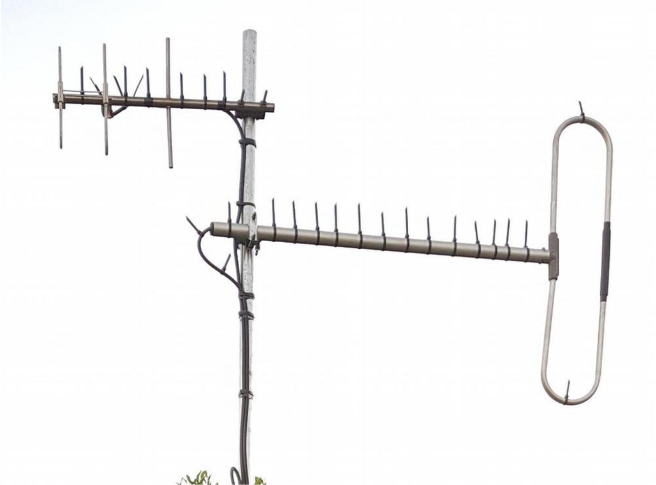
*Illustration 4: The antennae, complete with bird proofing.*
